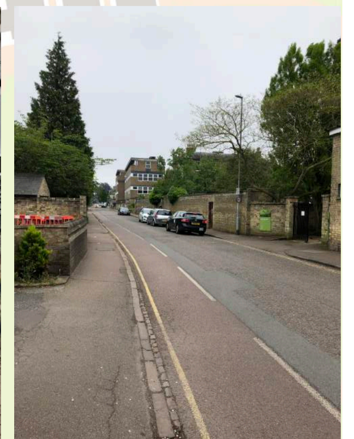
View of school from west end of Bateman Street
